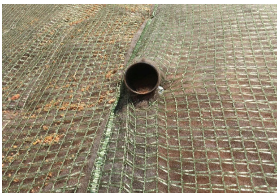
Figure 11. Installation of the drainage pipes [3]
