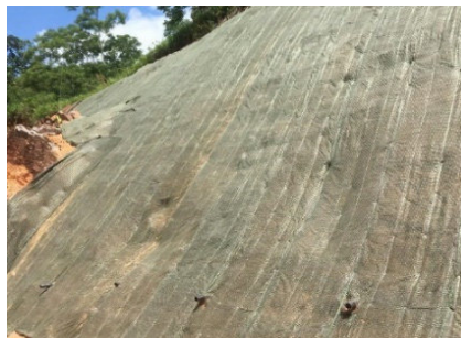
Figure 9. Installation of the drainage pipes [3]
