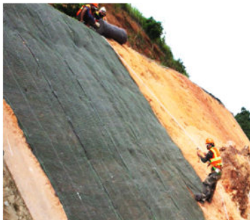
Figure 8. Installation of the Takino mat [3]
