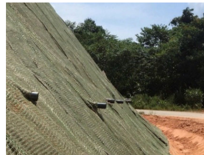
Figure 10. Installation of the drainage pipes [3]
